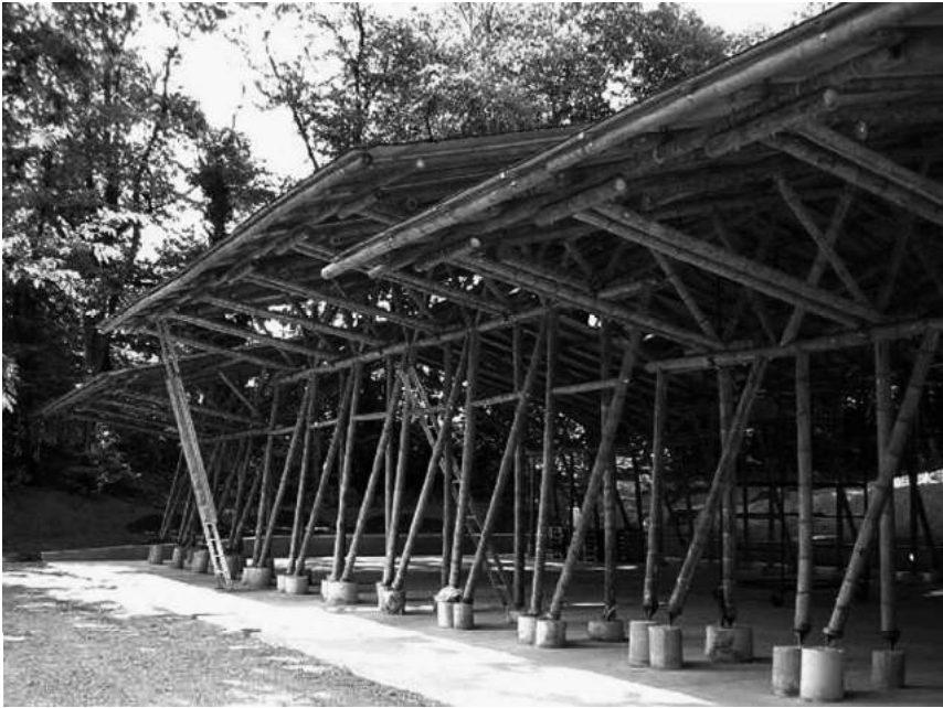
Figure 1. Side view of the building.
