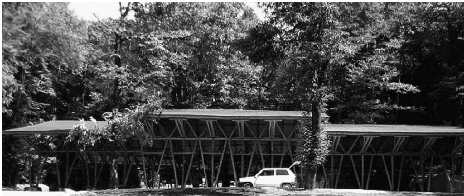
Figure 2. Front view of the building.
