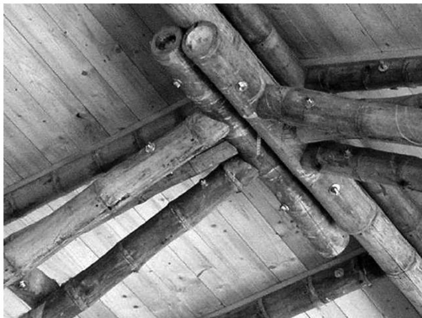
Figure 3. Detail of the roof.
